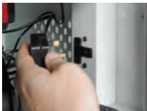
Each compartment is fitted with standard UK three-pin socket.
